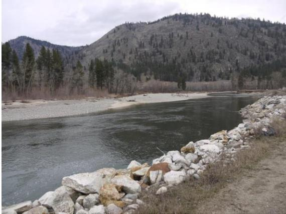
A stretch of the Kettle River that was filled with rock to prevent erosion but is now causing erosion downstream (Taken from Jenny Coleshill's presentation)
